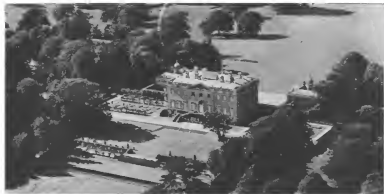
LEFT: The south front of Kirtlington Park. The grounds were landscaped by Lancelot “Capability” Brown between 1752 and 1756.
